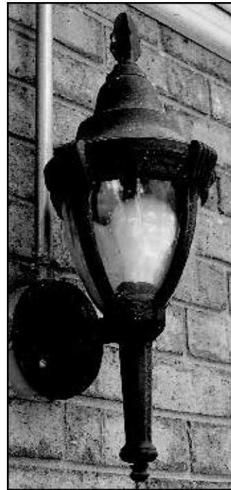
When installing outdoor security/decorative lighting, always follow local electric codes. This fixture uses rigid aluminum conduit. Photo by James Dulley.
